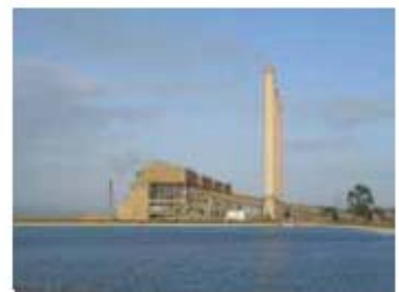
Hazelwood Power Station
